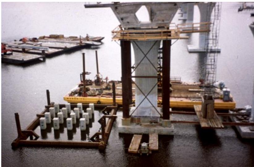
Figure D.2-2 Pile layout for pile group testing (from Anderson, 2015)
